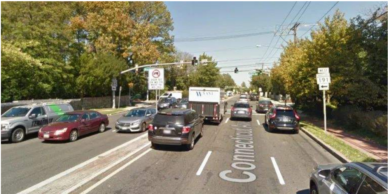
Figure 11. Example of narrow lanes on Maryland State Highway. MD 185 in Chevy Chase, MD. The general purpose lanes on this 30 mph arterial roadway are between 8 and 9 feet wide. Trucks are banned on this road.
