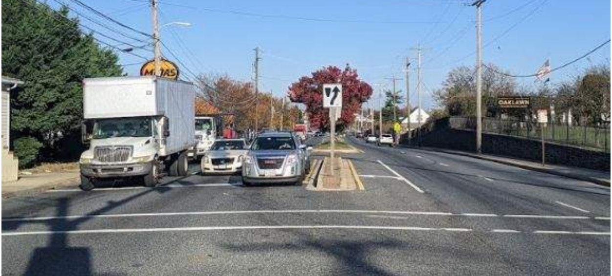
Figure 10. Example of narrow lanes on Maryland State Highway. MD 150 in Dundalk, MD. This 35 mph arterial roadway carries heavy truck traffic and has several intersections with 7-to-8 foot wide left-turn lanes.
