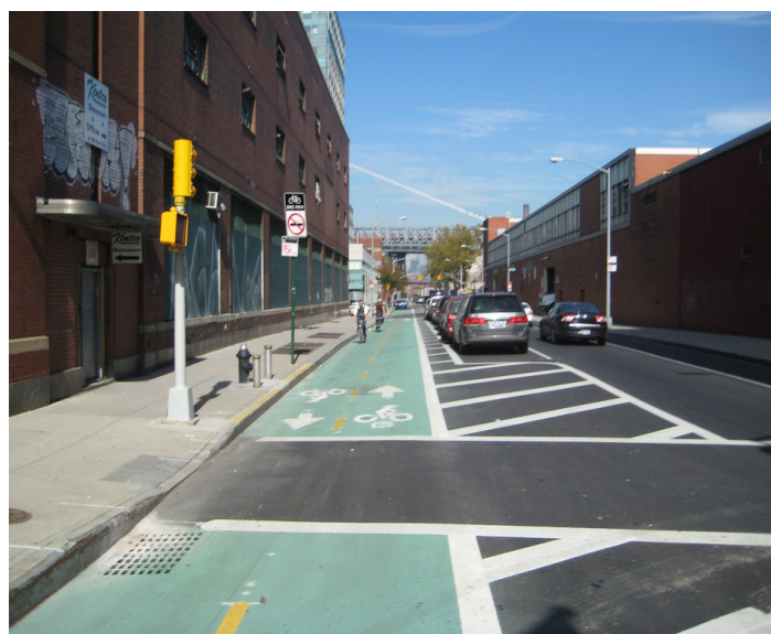
Use of colored pavement to designate a cycletrack.
