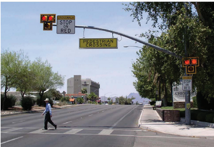
High-Intensity Activated crossWalk (HAWK)
