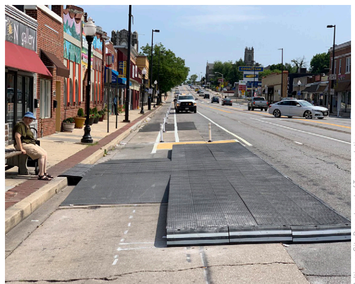
Floating Bus Stop on Harford Road
