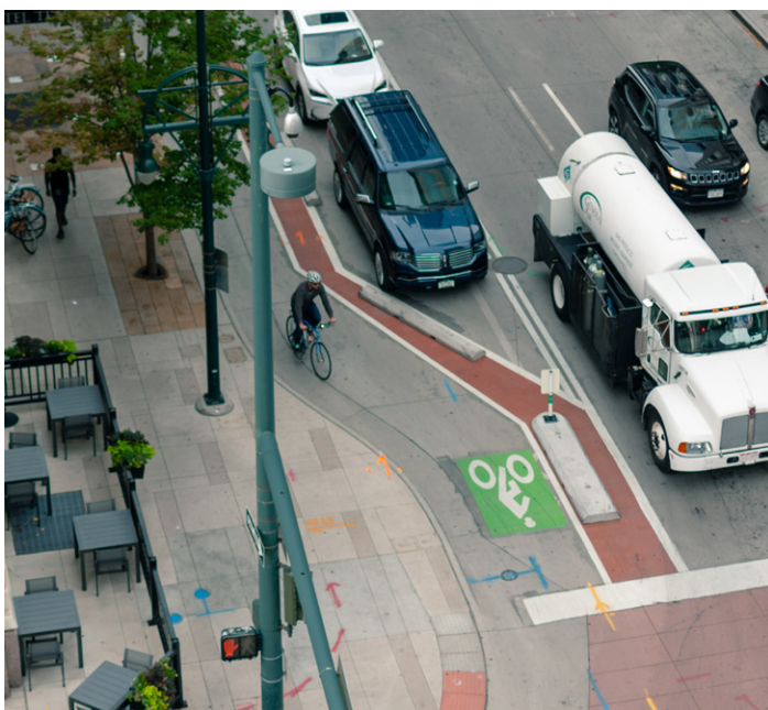
Separated Bike Lane Intersection Approach
