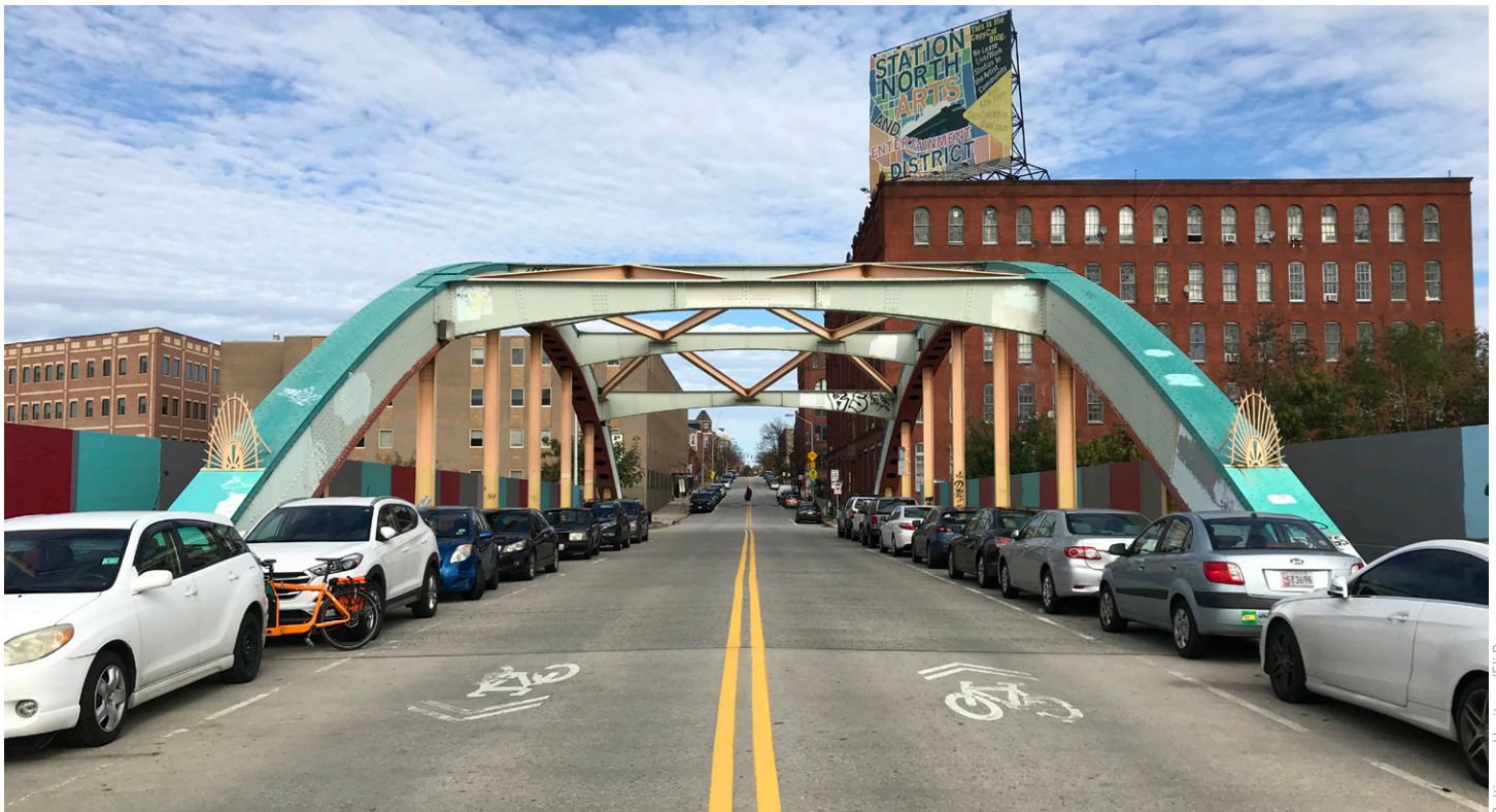
Guilford Avenue Bridge
