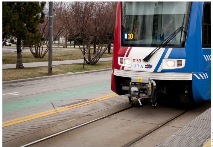
The use of rumble strips to separate light rail transit and bicycle lanes.
