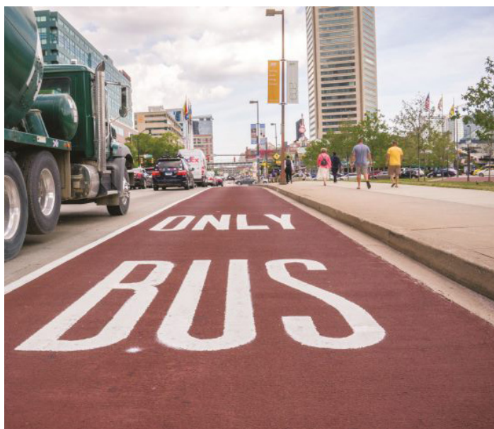
Bus Lane with Dark Red Paint on Pratt Street
