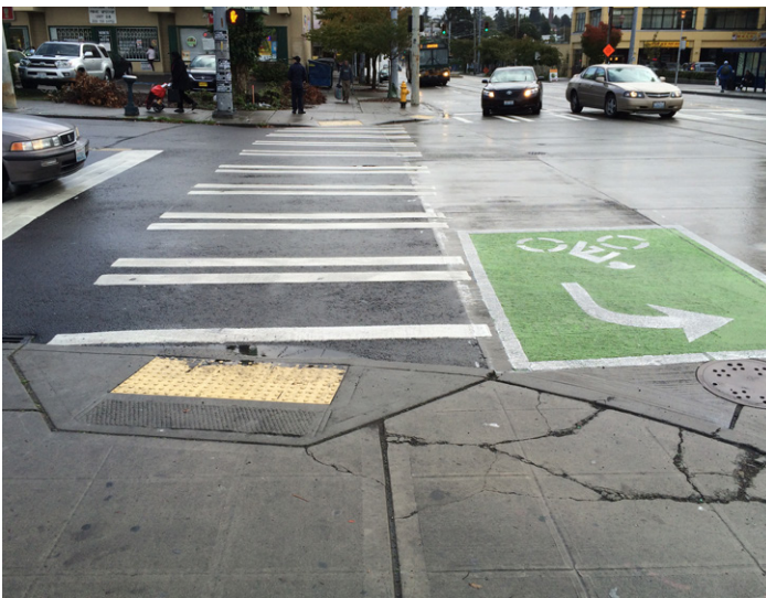
Two-Stage Left Bicycle Turn Queue Box
