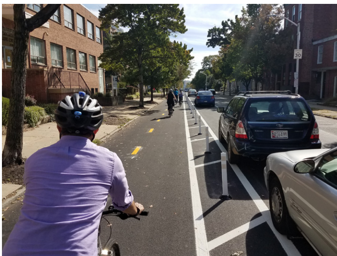
Maryland Avenue Separated Bike Lane
