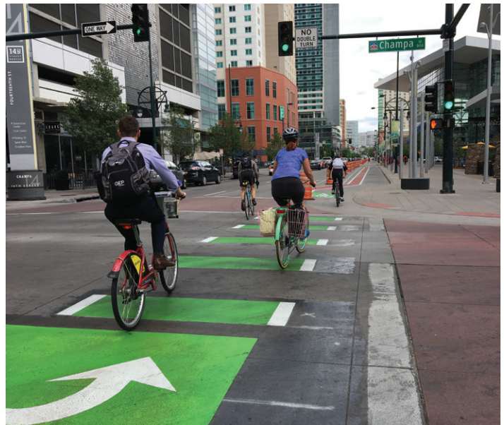
Green paint in bike lanes should be limited to conflict points with vehicles at intersections and high volume driveways.
