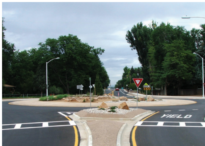
Roundabout with Mountable Apron
