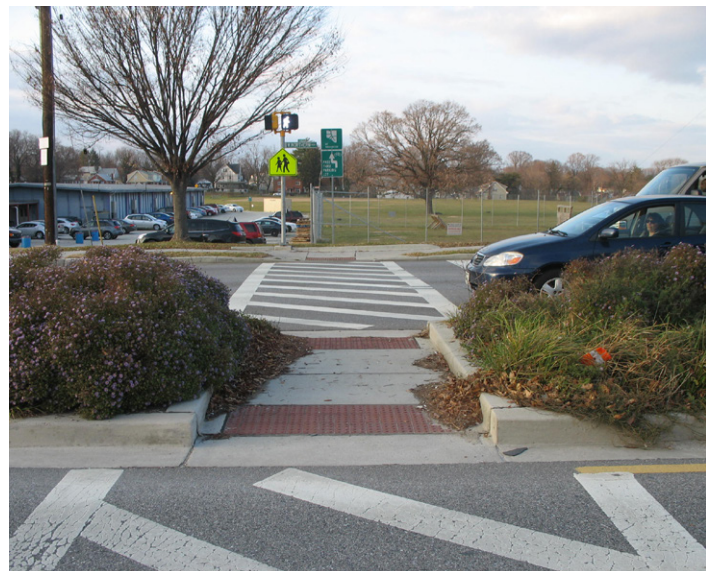
Pedestrian Safety Island on Northern Parkway
