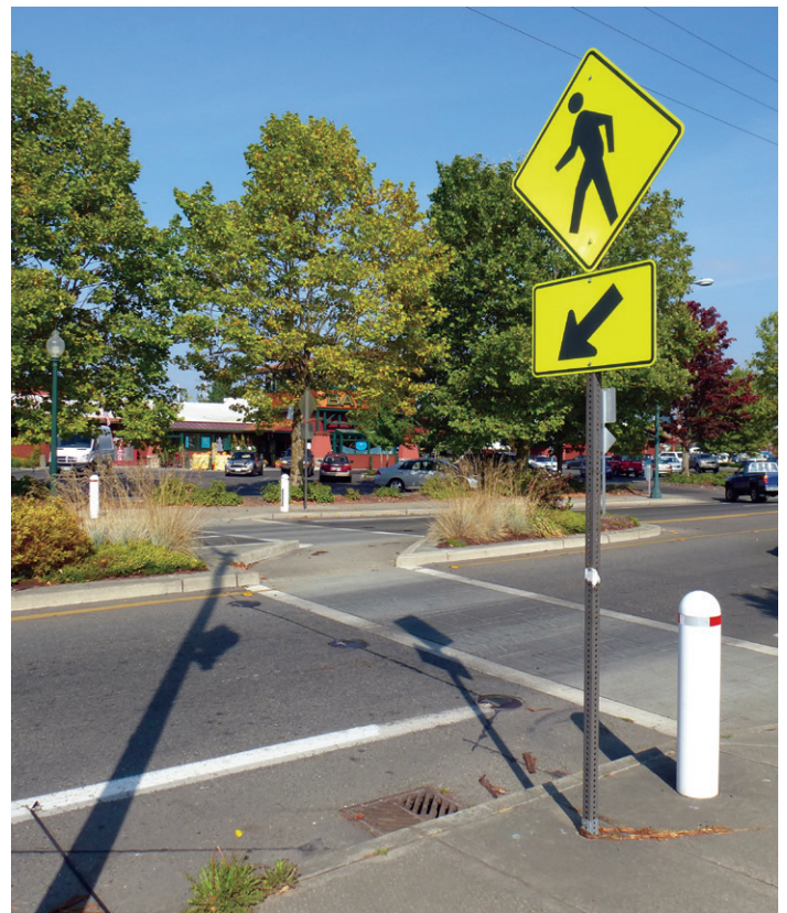
Raised Median with Pedestrian Safety Island
